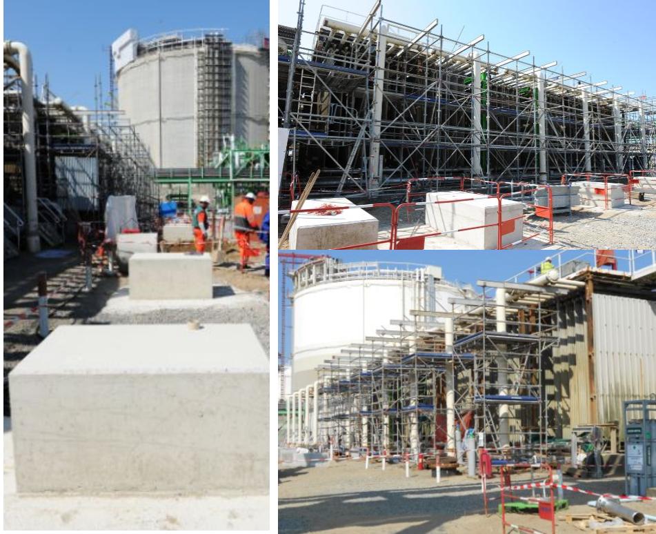
Figure 22: Typical works on ORV's supporting structures
