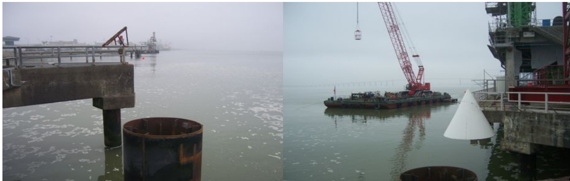
Figure 24: The existing pile is cut at its top
