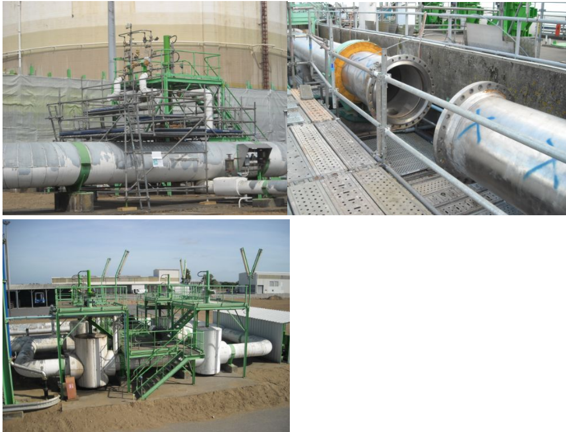
Figure 20: Typical works including cryogenic valves replacement
