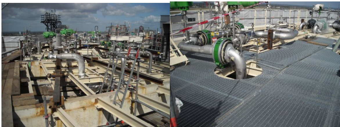
Figure 17: Typical works carried out on the dome
