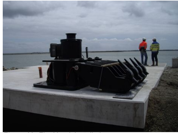
Figure 29: Final hook installation
