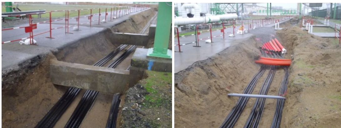
Figure 21: 6.6 kV cables replacement
