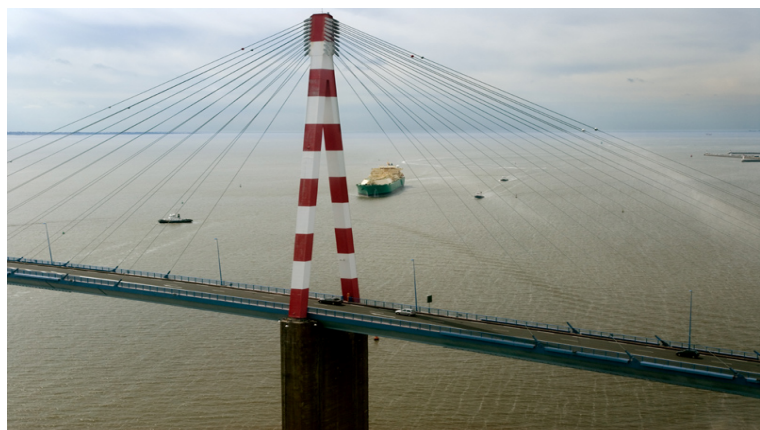
Figure 2: Port access overview
