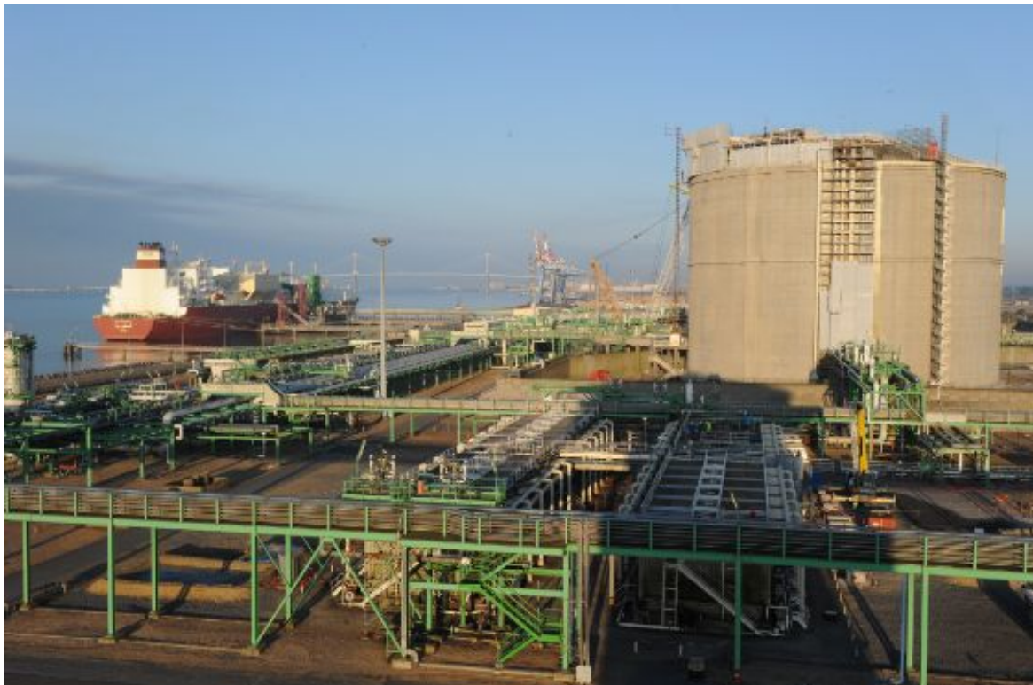
Figure 16: Tank overview before painting works
