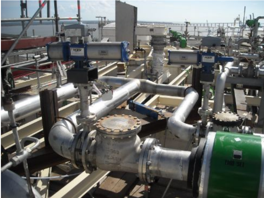
Figure 18: Valve replacement on the top of a tank
