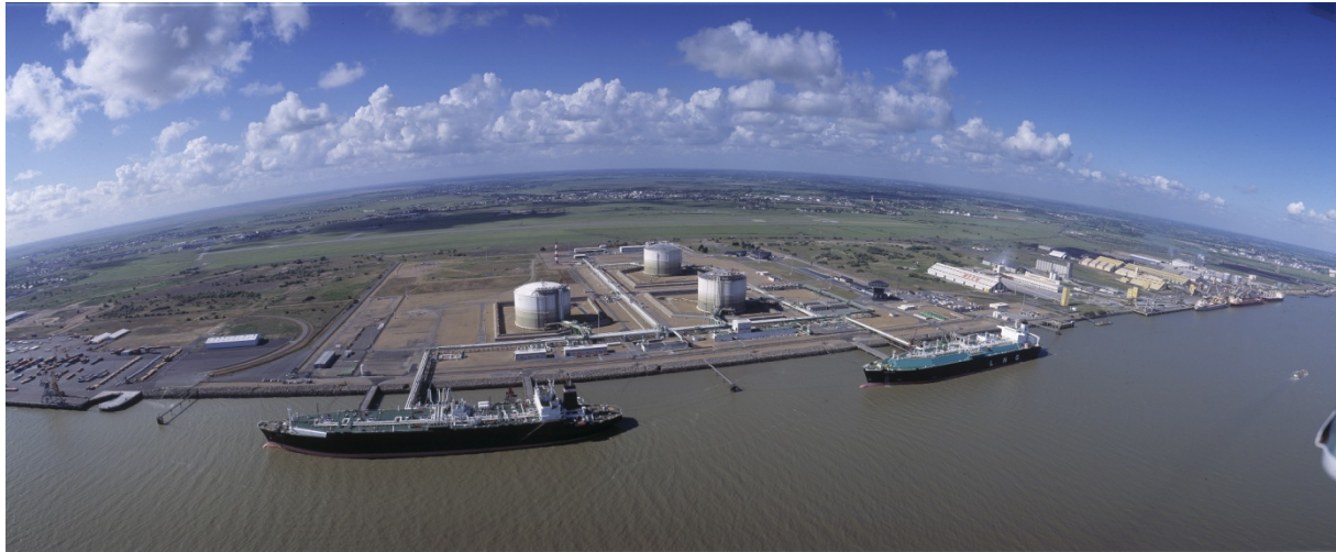
Figure 1: Terminal general layout highlighting the ability to receive two LNG Carriers
