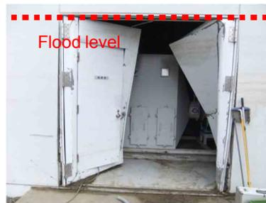
Fig. 6 Damaged Door
