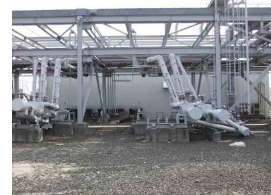
Fig. 9 Deformed Piping
