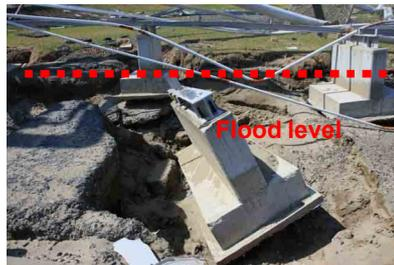
Fig. 8 Scouring of Piping Framework
