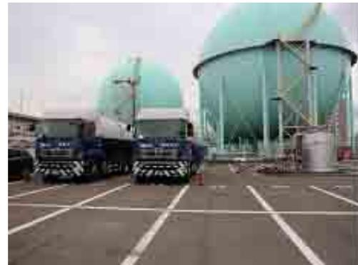
Fig. 15 Temporary LNG regasification equipment
