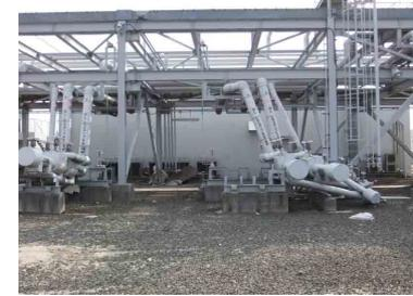
Fig. 9 Deformed Piping
