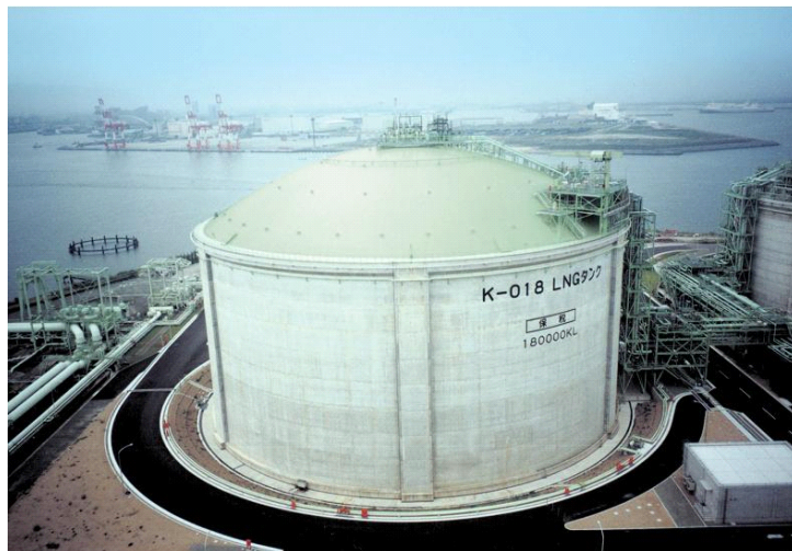
Figure 1 Appearance of 180Ml class LNG tank
