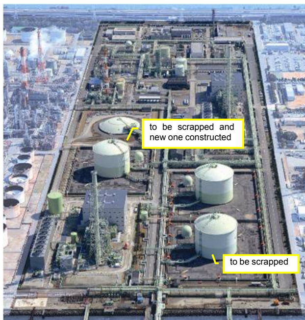
Figure 25 Senboku terminal 1 of Osaka Gas
