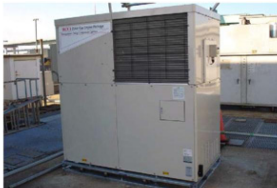
Fig.4 Newly developed 25 kW HCCI package
