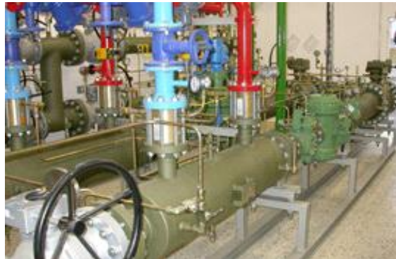
Figure 4.9 Pressure-regulating station
