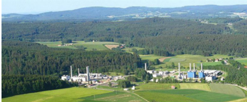
Figure 4.7 Compressor station in Germany with 8 compressor units
