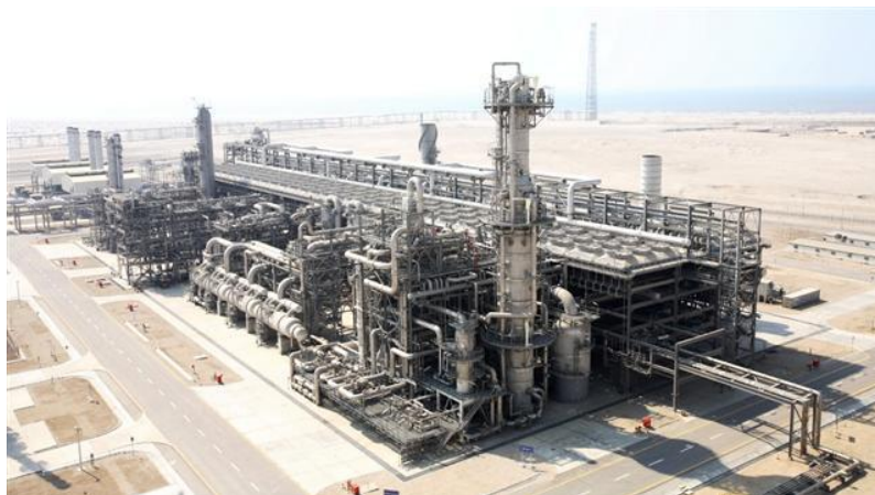
Figure 4.12 Liquefaction Plant – SEGAS, Damietta
