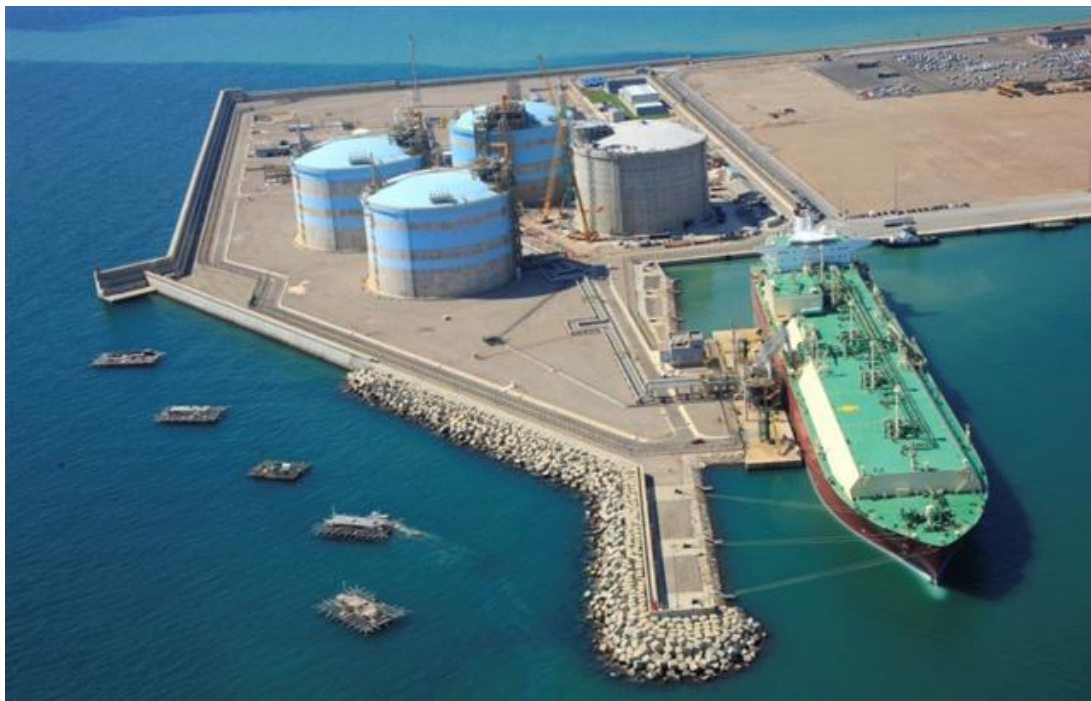
Figure 4.14 LNG receiving terminal
