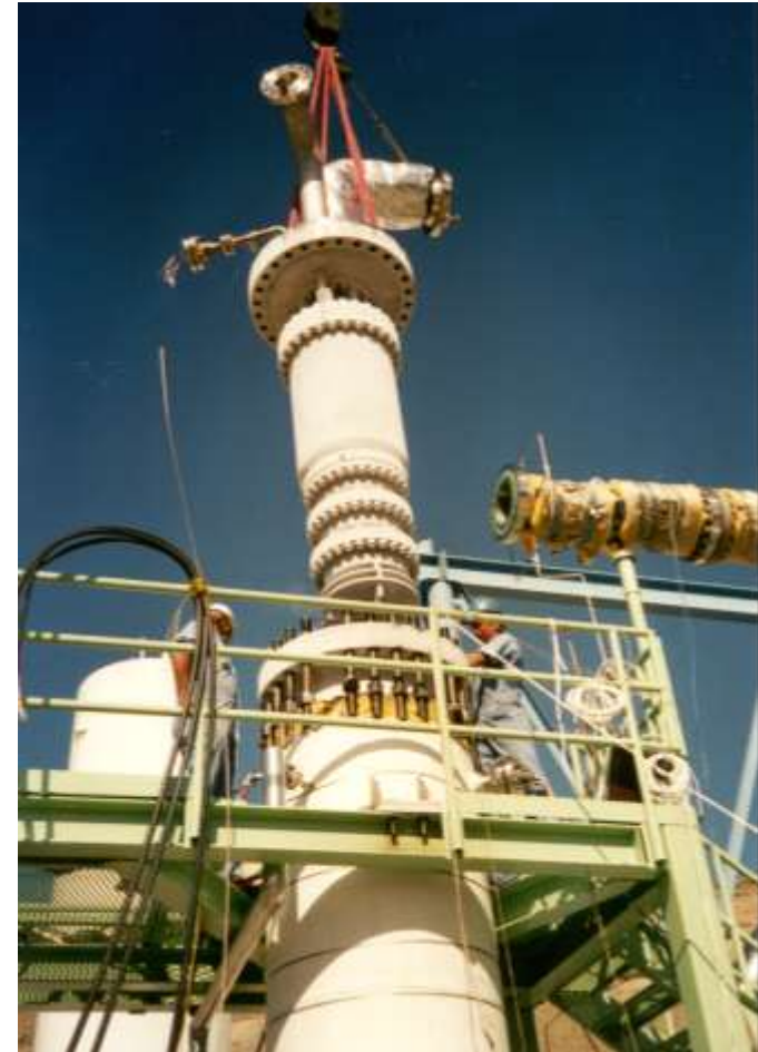
Cryogenic Liquid Expander Used by permission, Ebara International Corp.
