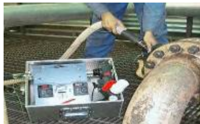
Oil and Gas Systems
