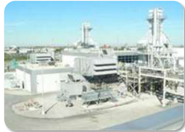
Two LM6000 aeroderivative gas turbines, above, power Toronto International Airport
