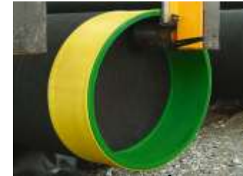
Inner Cap / Outer Cap assembly with spreader bar
