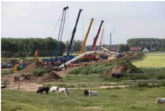
HDD – river Waal crossing NL
