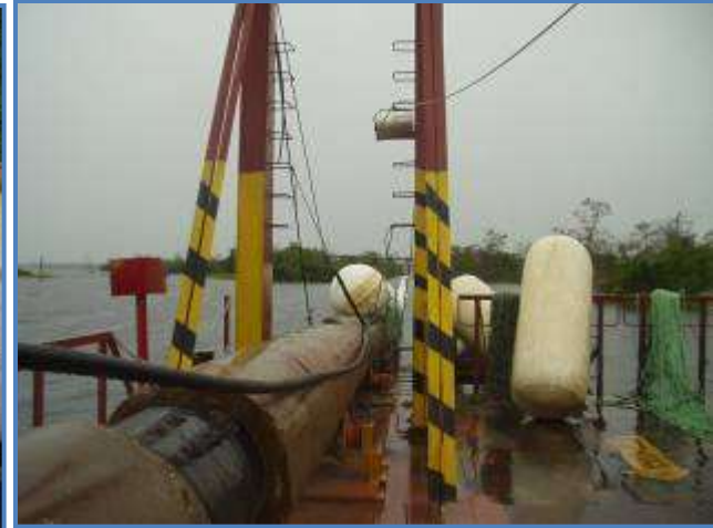
“PEAD” and float installation
