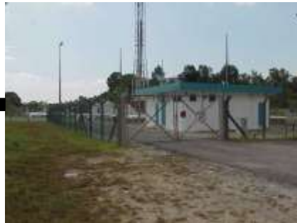
CITY GATE STATION
