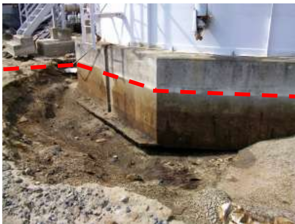
Water tank (pile foundation)
