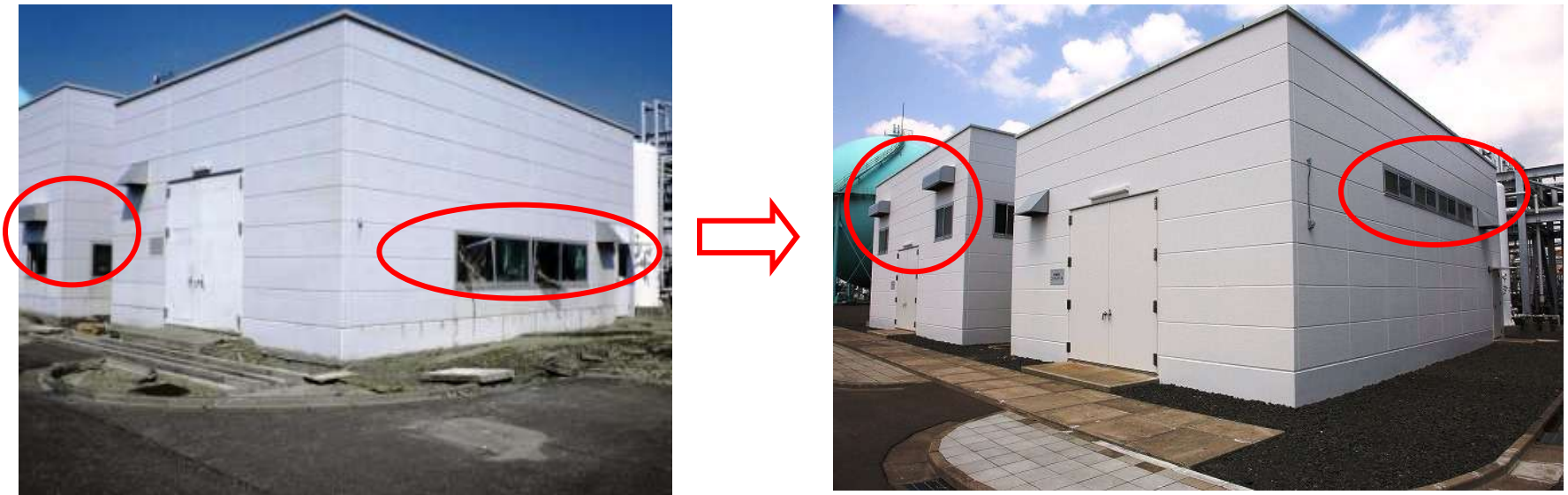
The Air compressor building
