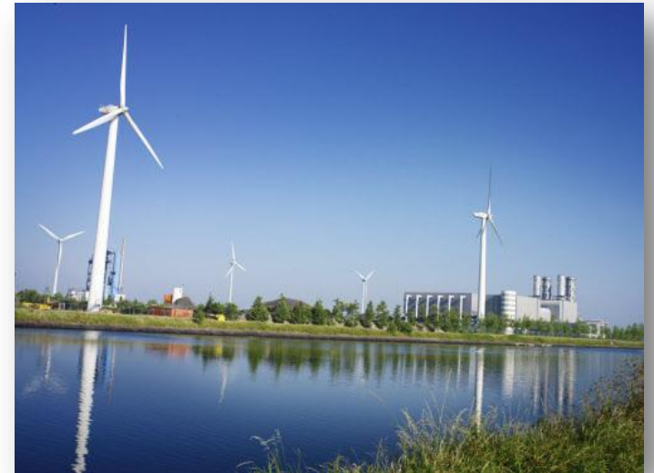
GDF SUEZ, CCGT Herdersbrug, Belgium
