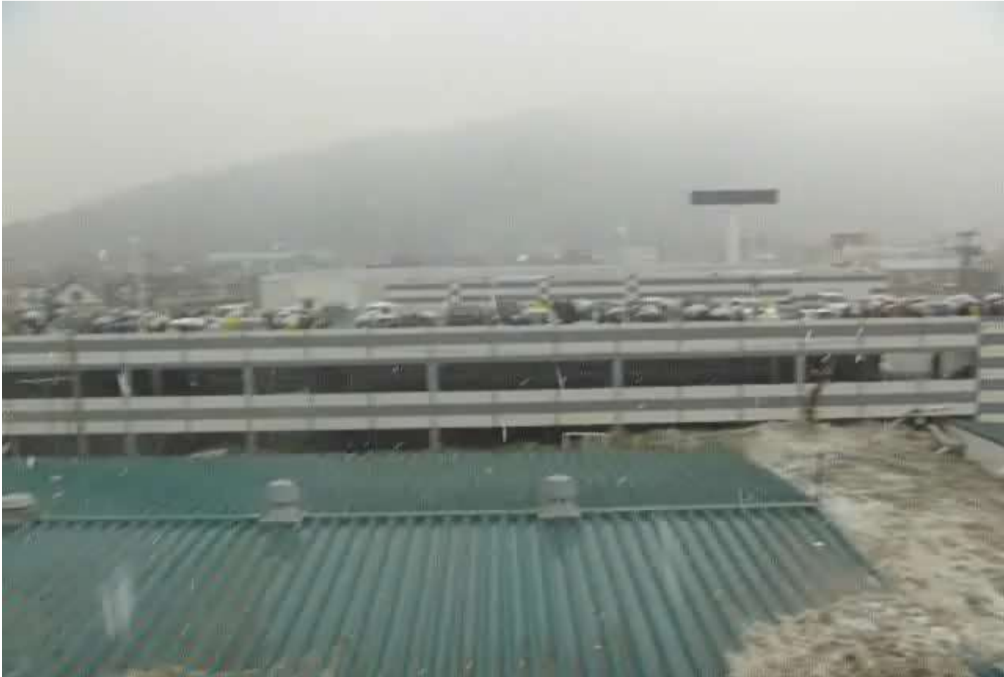
From top of the Ishinomaki Gas building © Ishinomaki Gas Co., Ltd.
