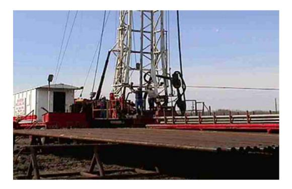
A "doghouse" is a small house located on the floor of an oil or gas rig that is usually used as an office or storage area
