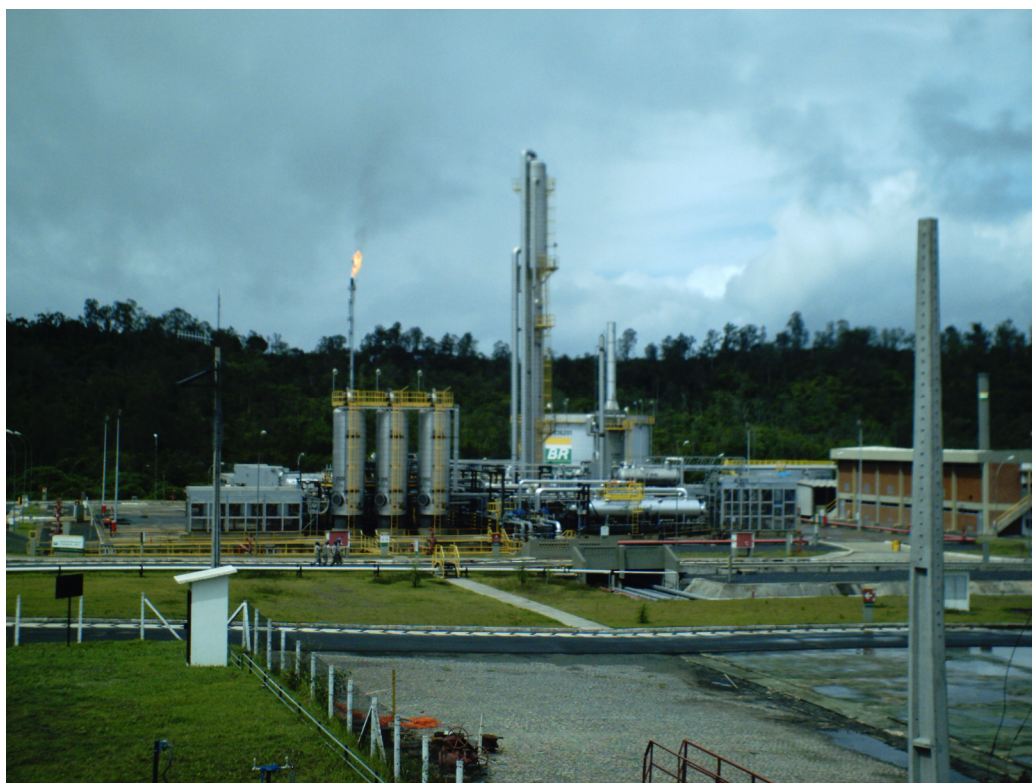
Figure 11 – Photo of the gas processing plant – Bahia, Brazil.
