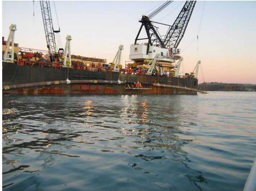
Figure 8: Last offshore pipeline weld – Algerian coast behind
