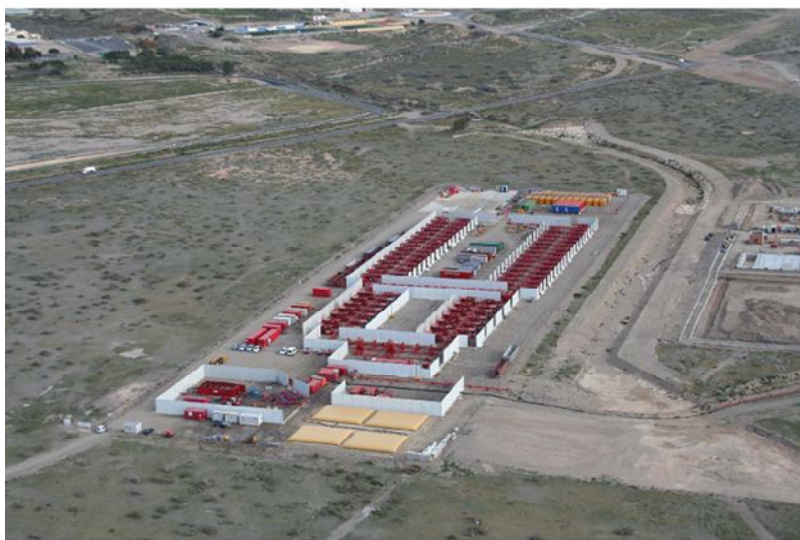
Figure 9: Temporary air compression facility during offshore construction and commissioning
