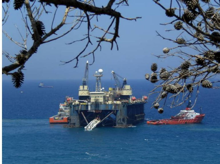
Figure 7: Pipe-lay operations - Algerian side
