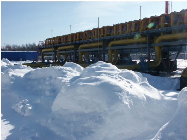
Fig. 12. Exterior view of ACU
