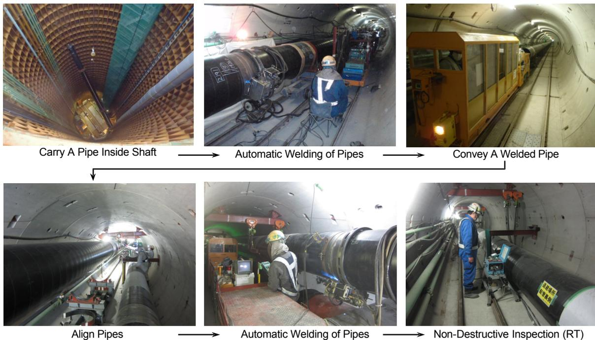
Picture 5 Site P photographs of Pipeline Installation Work inside Tunnel
