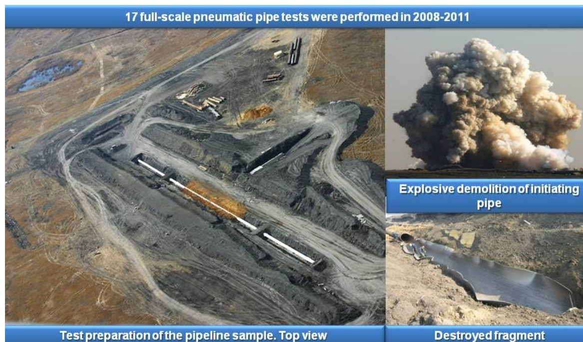
Fig.7 - Pneumatic field tests of X80 pipes, town of Kopeysk
