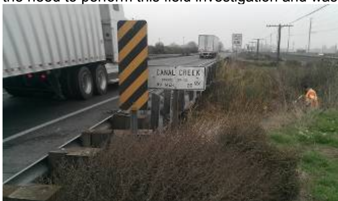
Figure 18. Field Excavation Example 1 (Image 1)
