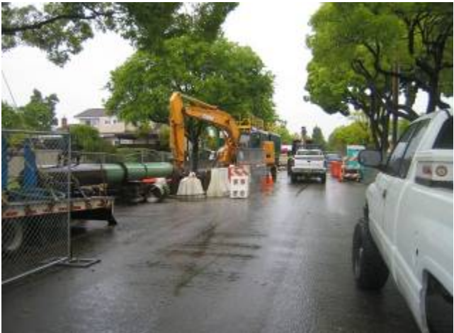
Figure 30. Hydrostatic testing in process
