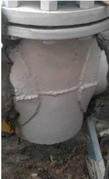
Figure 21. Field Excavation Example 1 (Image 3)
