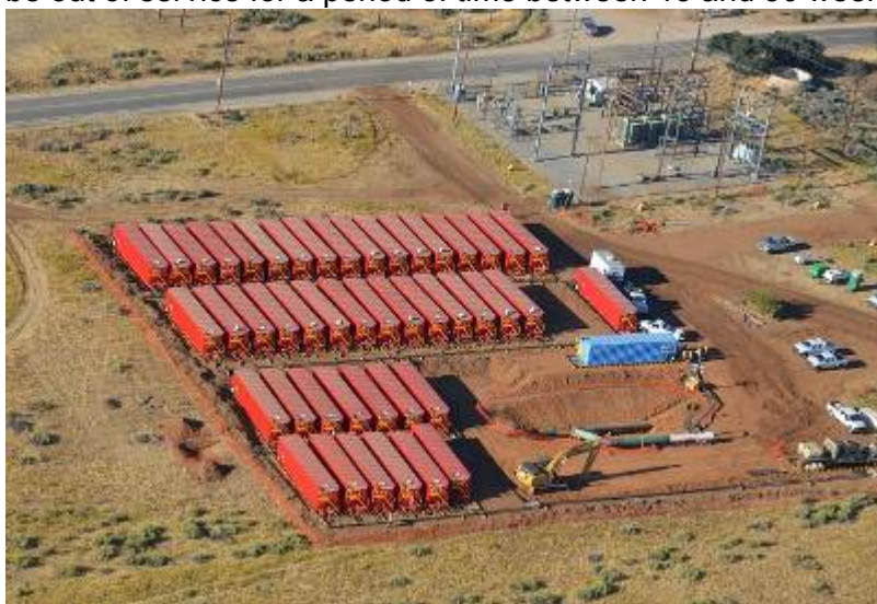
Figure 28. Hydrostatic Test Set up
