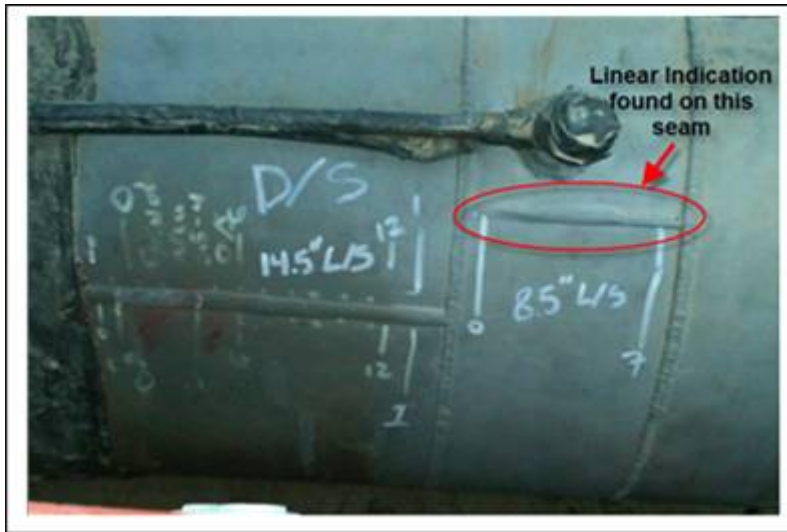
Figure 23. Field Excavation Example 2 (Image 2)
