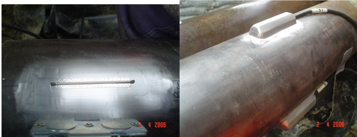
Figure 3: Strain Gages - Installation.
