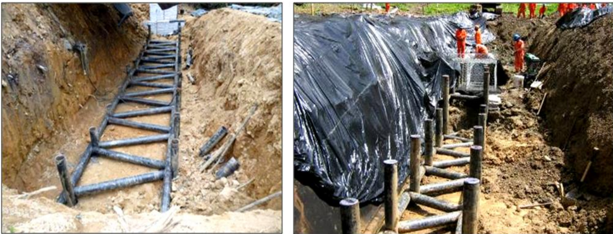
Figure 3-15 – Bracing of piles
