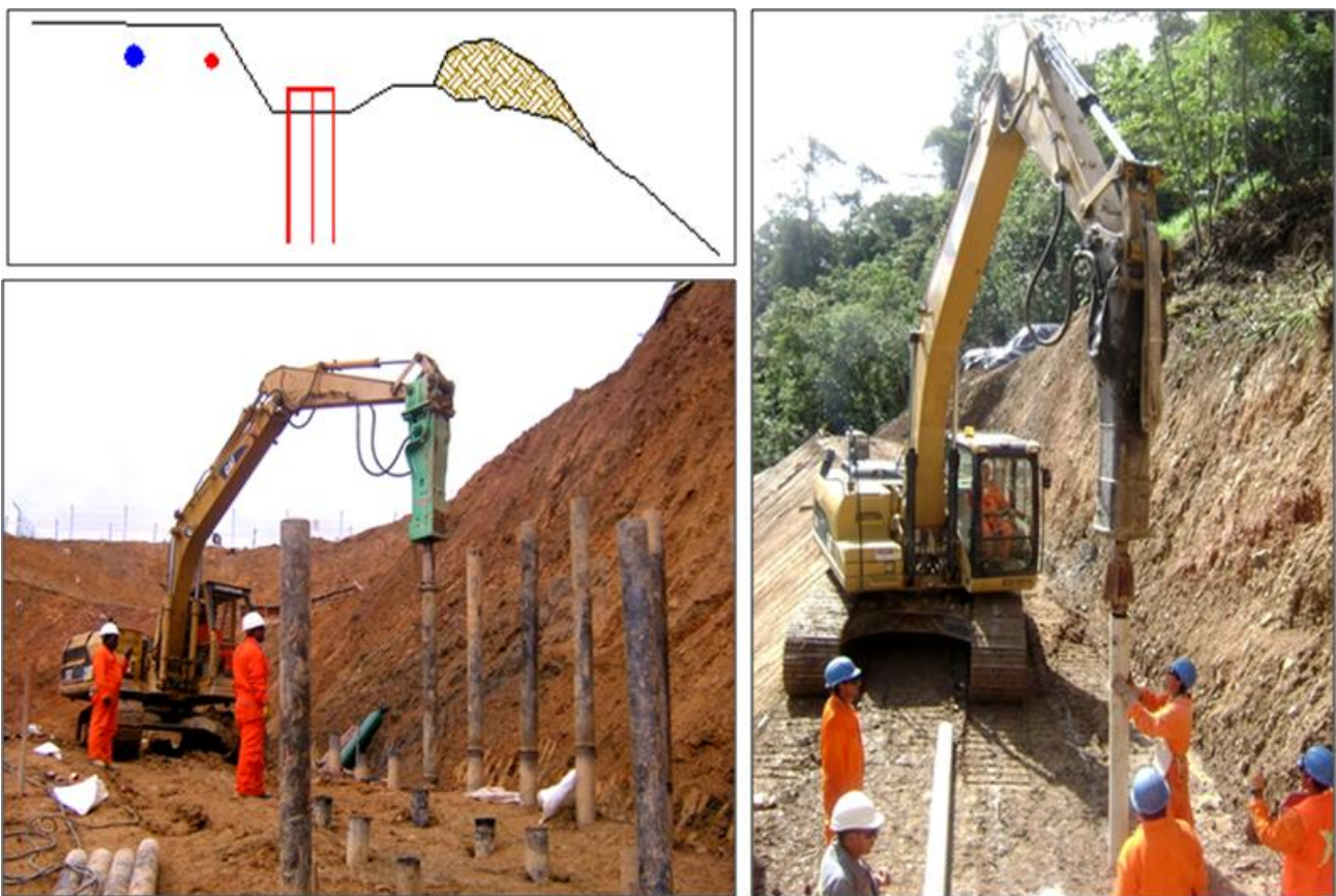
Figure 3-13 – Driving of piles
