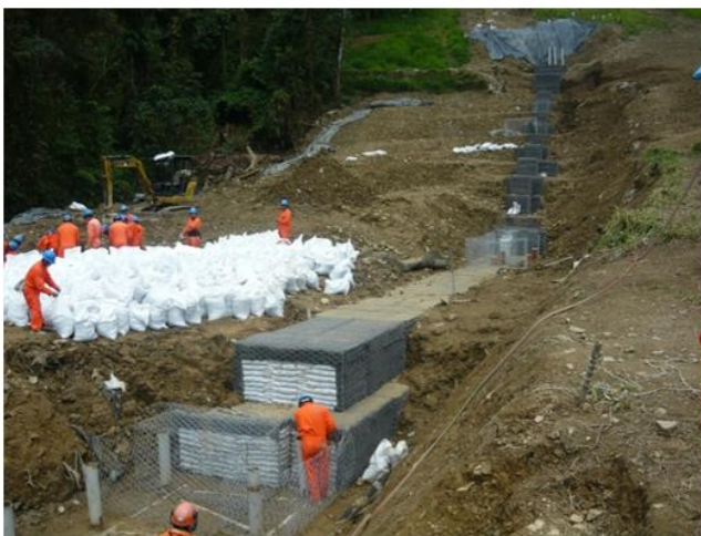
Figure 3-17 – Assembly and construction: next level of the gabion
