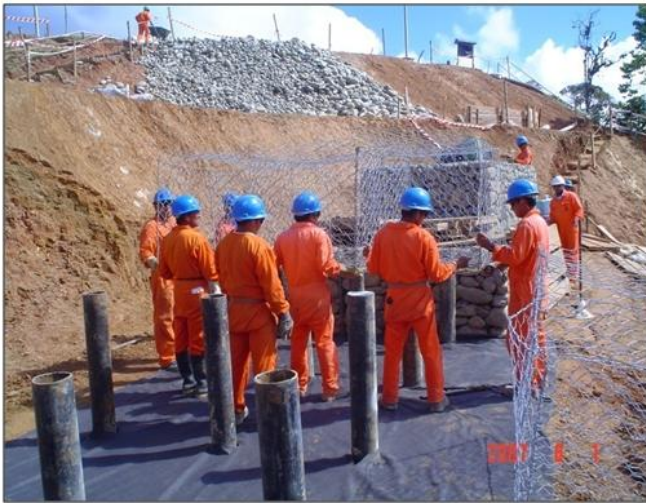
Figure 3-16 – Assembly and construction: first level of gabions
