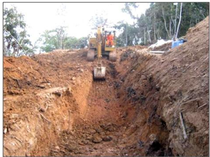
Figure 3-11 Excavation for the driving of piles
