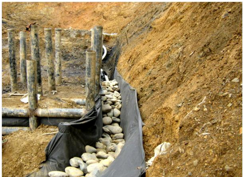
Figure 3-12 Construction of filters
