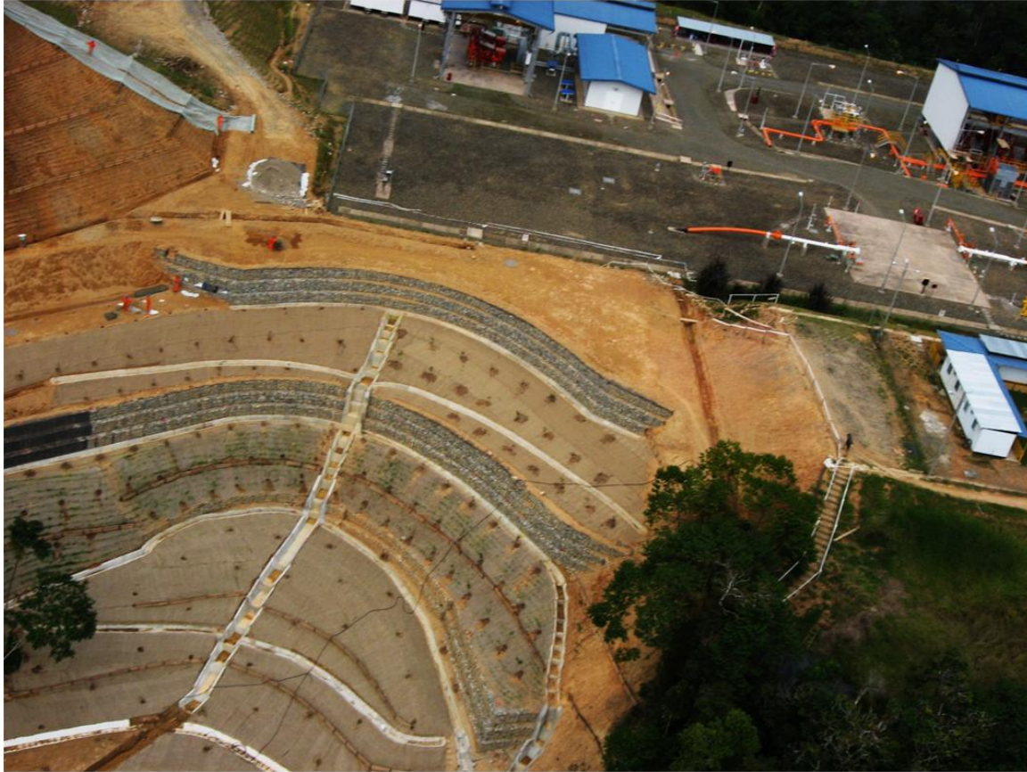
Figure 3-18 – General view of the completed work
