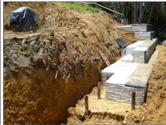
Figure 3-16 – Assembly and construction: first level of gabions
