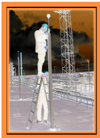
Figures 4a, 4b – Inspection of surface equipment, detection of leaks
