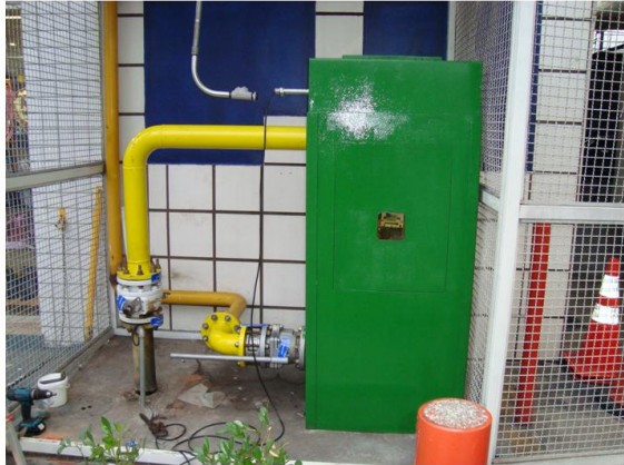
NGV Station A: after (meter with PU and with the box)
