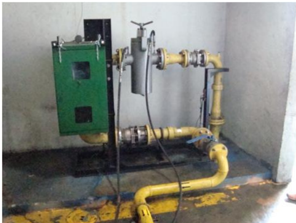
By pass at the filter pressure gauges positions
