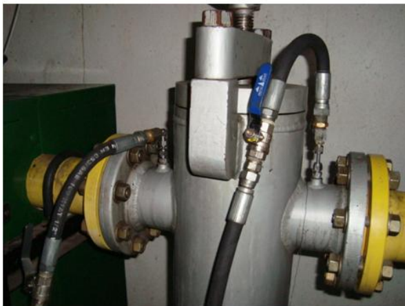
By pass at the filter pressure gauges positions
