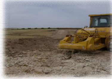
Works of opening of trench for the pose (installation) of the gas main Medgaz (Chentouf W Temouchent (Cosider-Sonatrach, Algeria) damaging a gas main with nearness emergency intervention.
