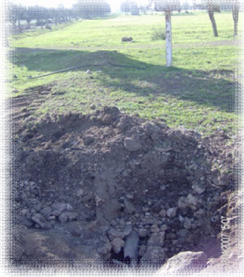
Agricultural works to Hassi-Bounif (W. Oran, Algeria) damaging a gas main in spite of the controls and the advice of the operators.
