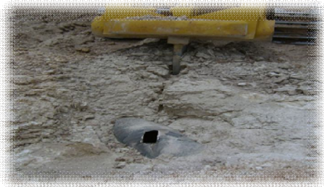
Works of opening of trench for the pose (installation) of the gas main Medgaz (Chentouf W Temouchent (Cosider-Sonatrach, Algeria) damaging a gas main with nearness emergency intervention.
