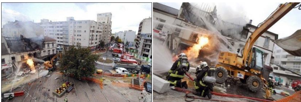
Bondy (30-10-2007) - Perforing of a pipe and a breach(negligence) in an obligation(bond) of caution, explosion and fire, 1 deaths, 63 wounded persons among whom 10 brulés (Paris region, France)
