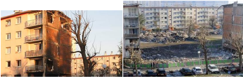
Noisy-le-Sec (22-12-2007) - Gas leak and explosion further to works of drilling. Building HLM(COUNCIL HOUSE) STEPHENSON destroys by the explosion, those adjoining very damaged ( 76 impacted households. 176 mobilized fire brigades - (Noisy-le-Sec, Paris region, France)
