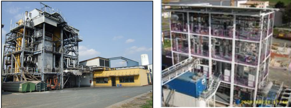
Fig 13: Repotec FICFB gasification process – Güssing cogeneration units and méthanation pilot plant
