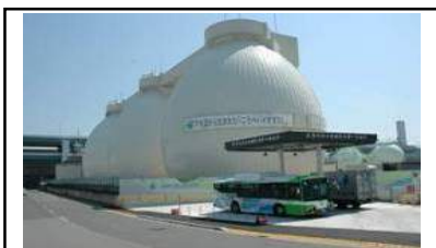
Picture 3 Biogas Station
