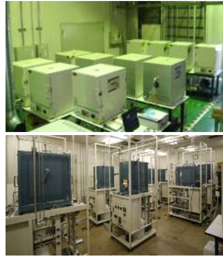
Figure 7. Experimental facilities (Osaka Gas)
