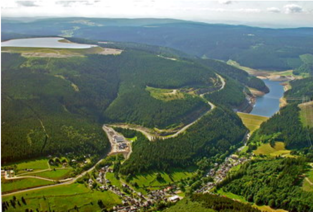
Figure 2 Pump-storage plant Goldisthal, Germany, 1060 MW, 8 hrs
