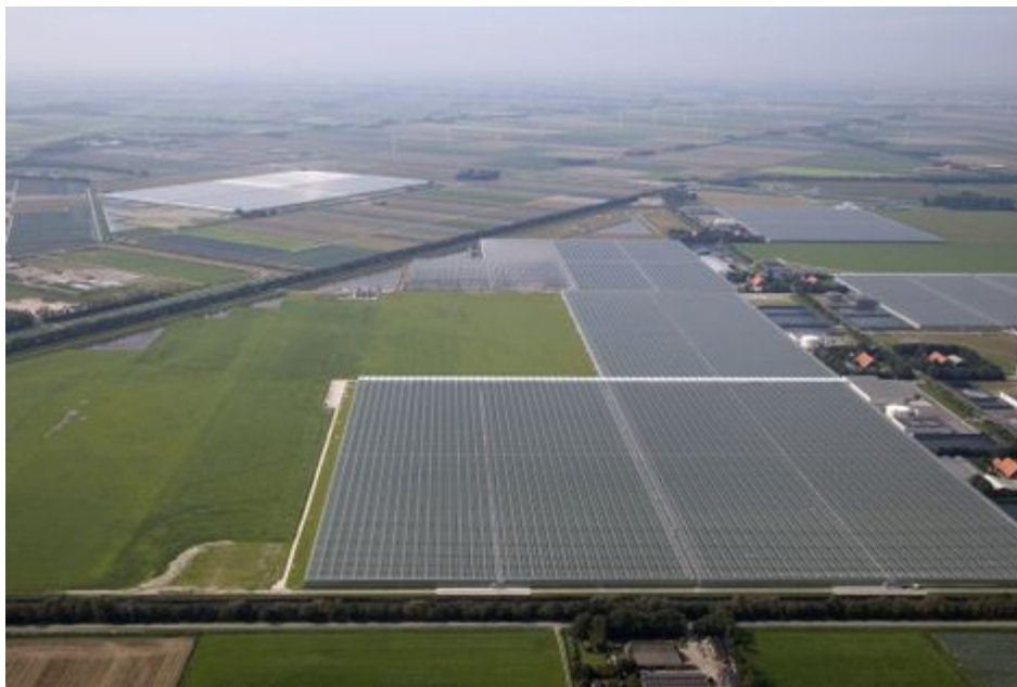
Figure 11, Greenhouses with CHP, supplying electricity, heat and CO 2 . Heat storage in white tanks on right hand side.
