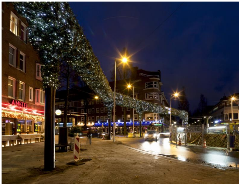
Image - The project team was forced to reroute a sewage pipeline above ground to continue drilling. The sewage pipe would be extremely visible and go over a square and past a restaurant. The project team invested in decorations, making it a trail of green and light instead of a big nuisance.
