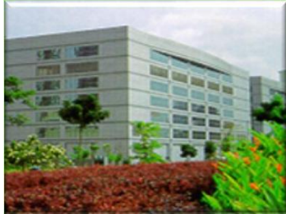
Fuel for Gas District Cooling
