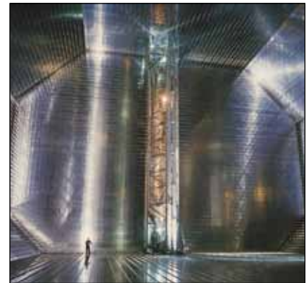
Inside a GTT membrane tank.
