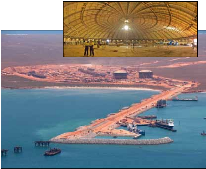
▲ Gorgon LNG's liquefaction plant is being built on Barrow Island. INSET Inside one of the plant's LNG storage tanks.
