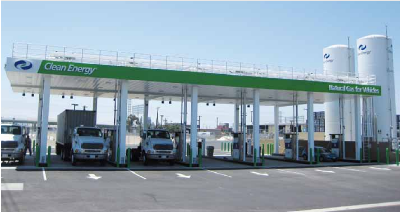
▲ The Clean Energy Fuels public CNG/LNG fuelling station in Long Beach, California. A well-rounded fuelling station network is evolving throughout the US and Canada.
