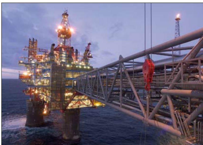
Carbon capture and storage has been carried out at the Sleipner Vest field since 1996.
