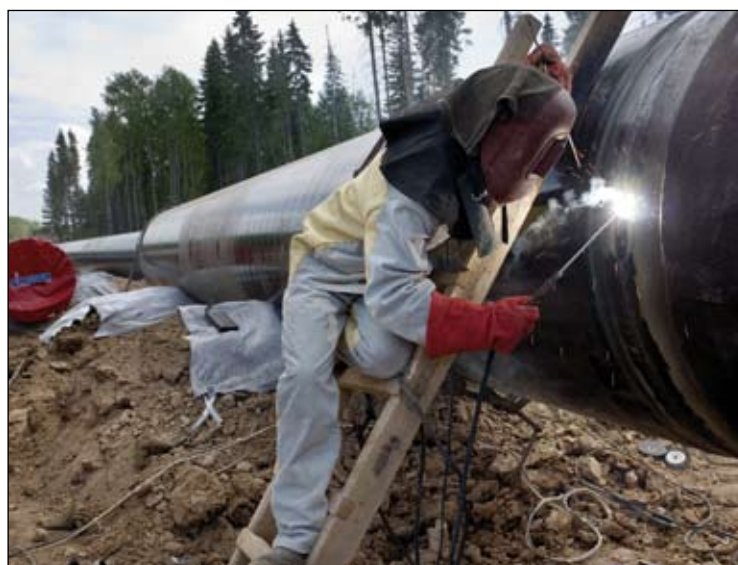
Laying the onshore section of Nord Stream.
