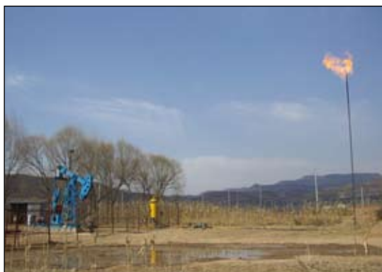
A CBM well in Jincheng, Shanxi Province, China. Utilising multi-lateral drilling techniques has made the well 40 times more productive than vertical drilled wells in the region.
