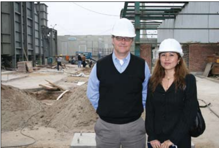
Sudamericana de Fibras (SdF) became the first company in Peru to use natural gas from the Camisea field for cogeneration in July 2006 and recently developed a second and much larger cogeneration plant. On site in the picture are Enrique Gubbins, General Manager of SdF, and Katharine Fierro, Country Manager – WADE Peru.
