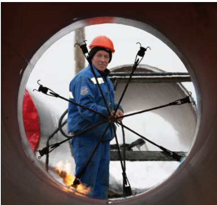
New pipelines are needed to bring gas to the European market.
