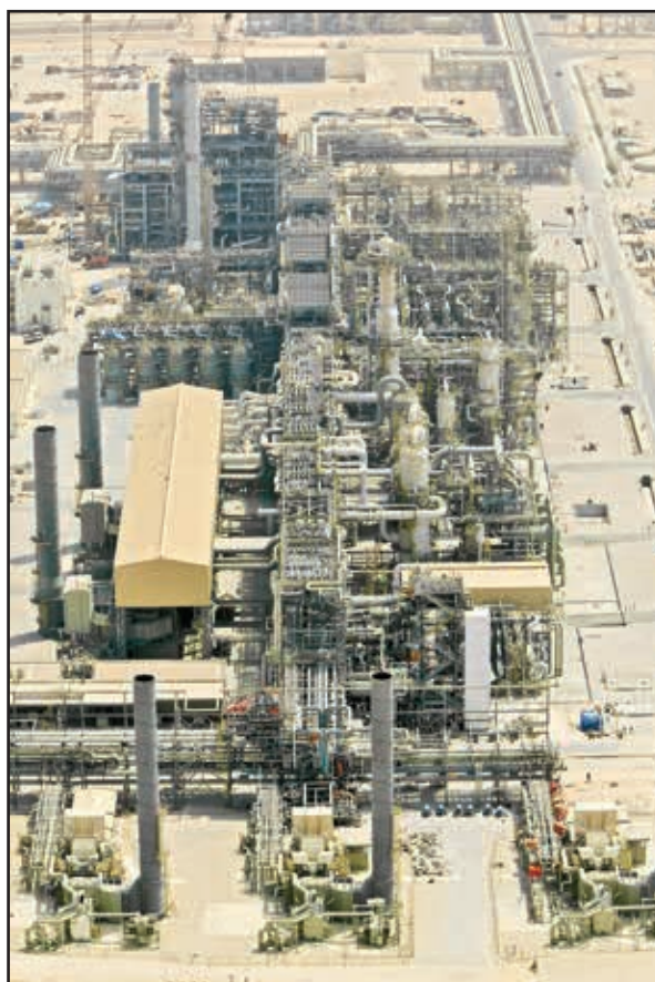
Train 4 was constructed with an excellent safety record.
