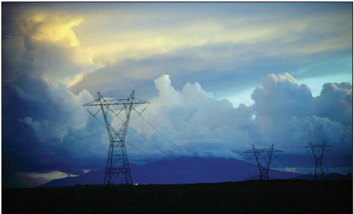
The challenge in meeting surging worldwide demand for electricity is less one of generation capacity and more an issue of grid capacity.
