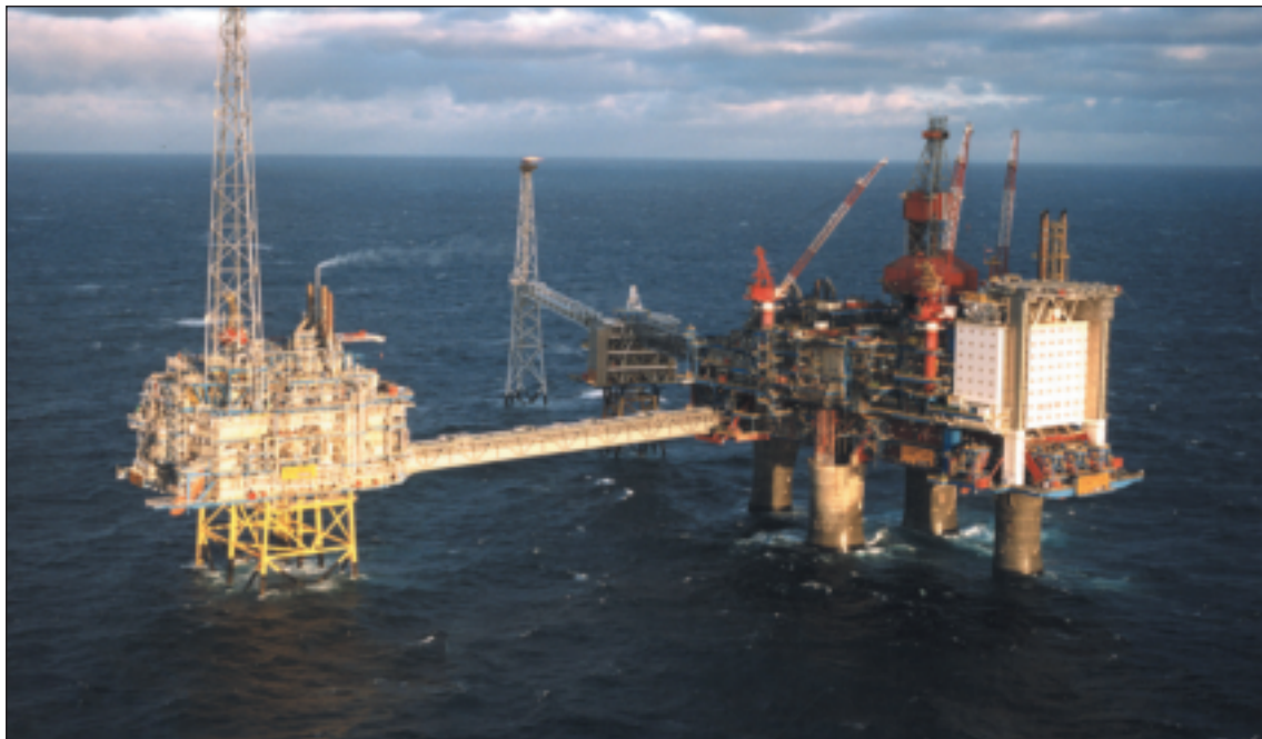
ABOVE AND OPPOSITE Natural gas in the Sleipner West field in the Norwegian sector of the North Sea has a 9% CO 2 content while its export specification calls for a maximum content of 2.5%. The excess CO 2 is extracted, compressed and injected into a saline aquifer.
