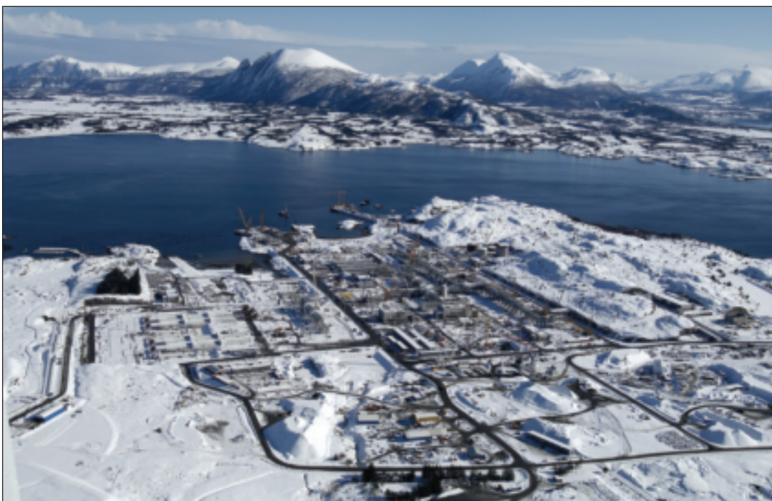
The Arctic region has already seen the discovery of giant gas fields such as Ormen Lange whose gas processing plant at Nyhamna is pictured.
