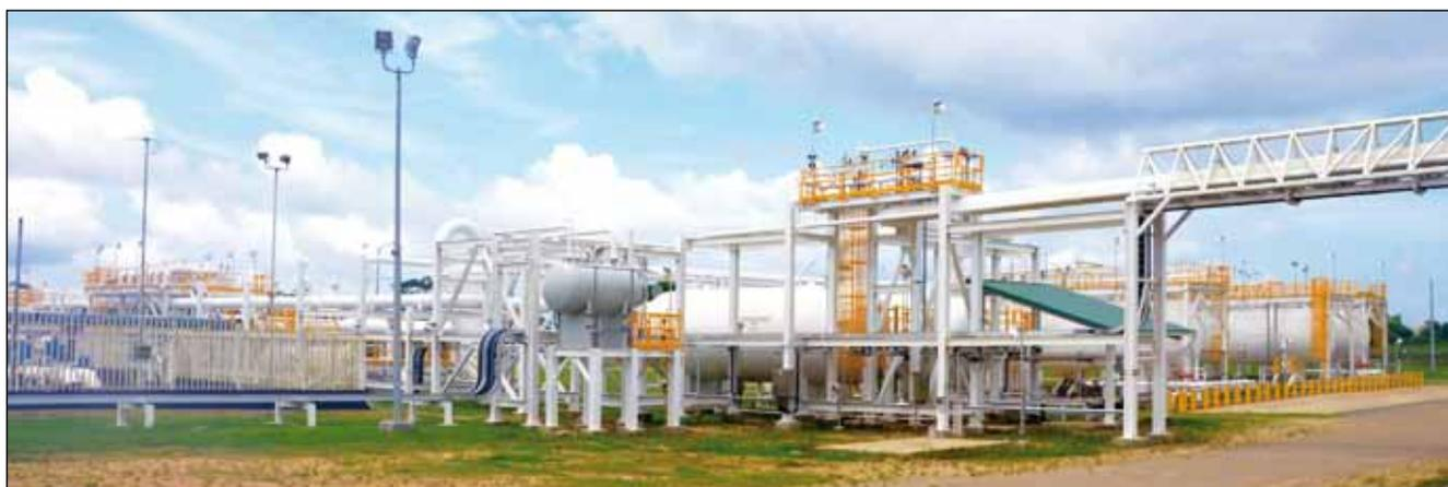
The Phoenix Park Valve Station, located at the Point Lisas Industrial Estate in Couva, is designed for the collection and distribution of natural gas and is a critical facility in NGC's pipeline system.
