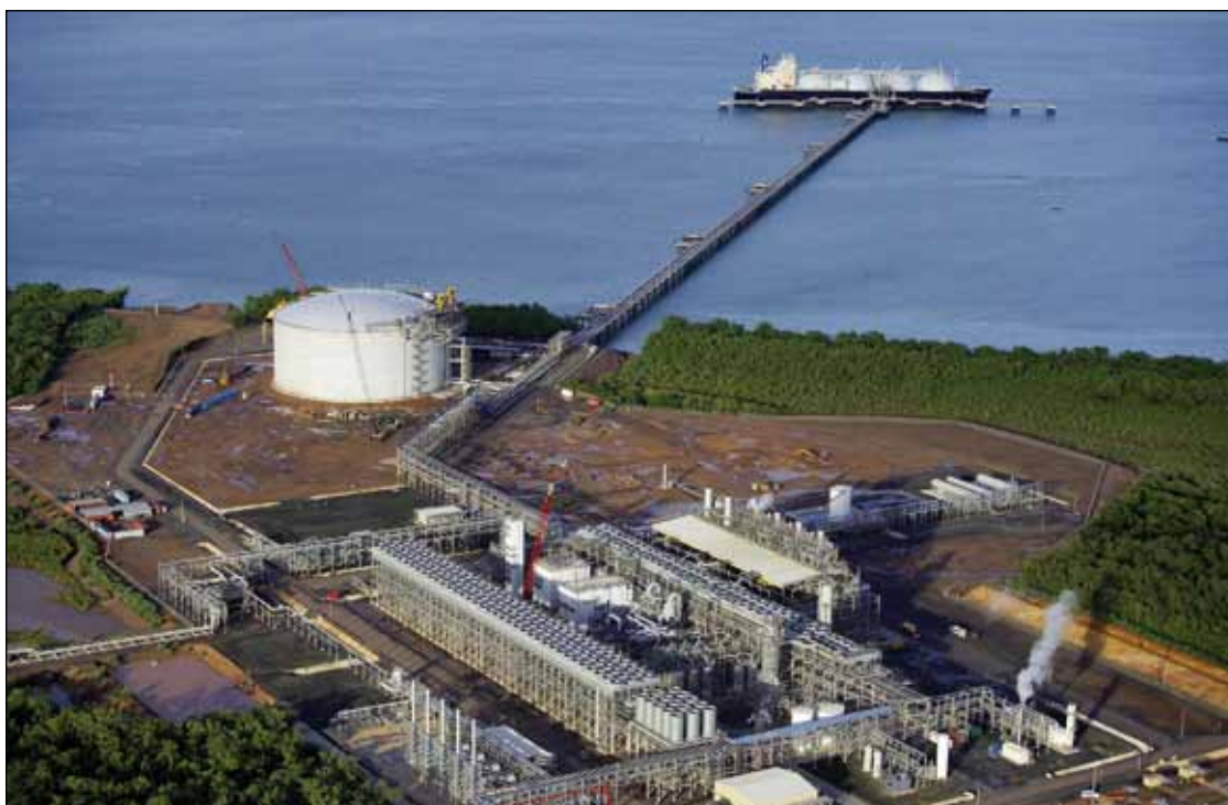
Darwin LNG was the first LNG plant to use aero-derivative gas turbines and started exports in February 2006.
