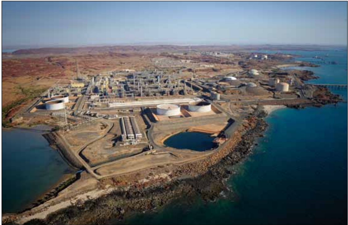
The North West Shelf venture began LNG exports in 1989 with two trains and now there are five with a combined capacity of 16.3 mtpa.
