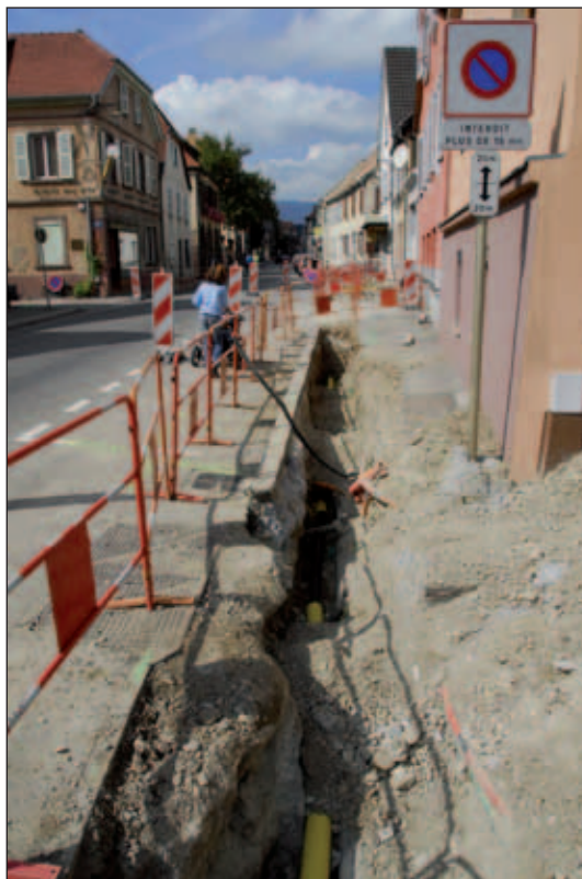
It is important to minimise the disruption caused by street works.
