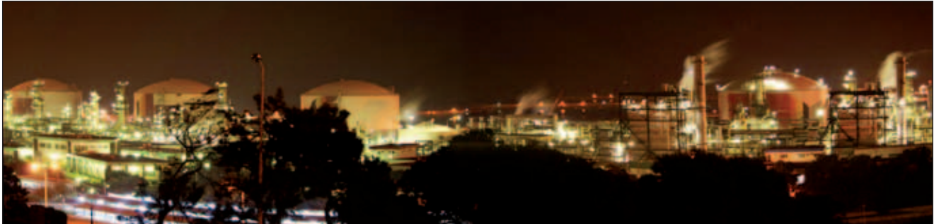
Sonatrach operates three LNG plants around Arzew – this is GL1Z – and one at Skikda.
