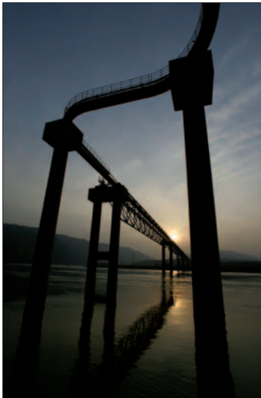
Pipelines such as the West-East in China are the core component to delivering the value and impact of natural gas.
