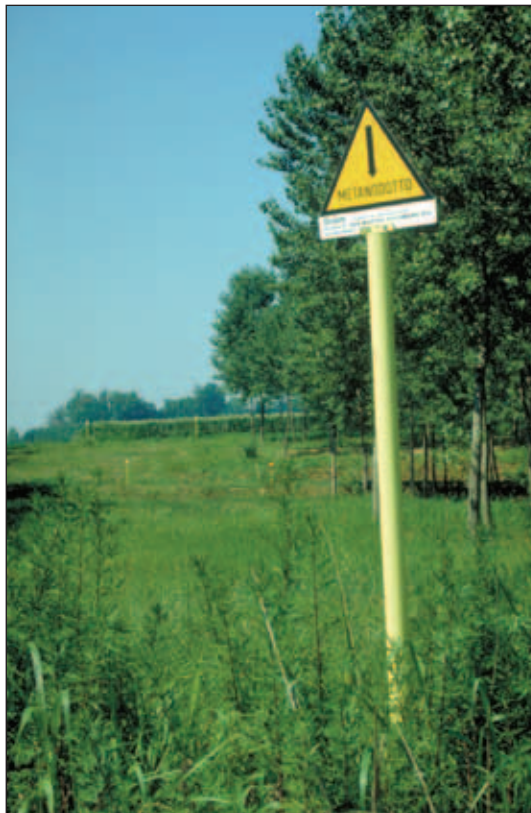
Route markers for a gas pipeline in Italy – pipelines operate in right-of-ways across property typically owned by others.
