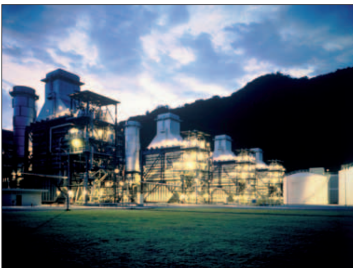
Thailand is one of the biggest gas consumers in ASEAN – a gas-fired power station in Khanom.
