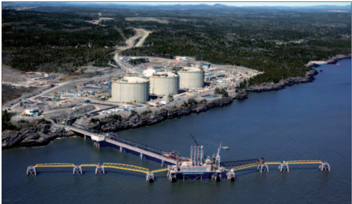
Canaport, Canada's first LNG receiving terminal, started up in June 2009.
