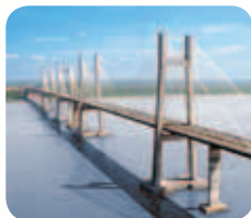
Second bridge spanning the Orinoco River Venezuela
