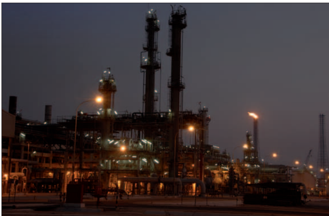
Qatargas 1 was designed to supply LNG with a high heat value to the Japanese market.
