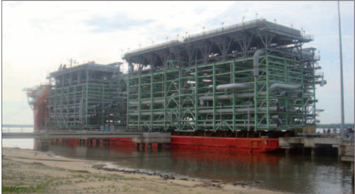
A delivery of components to the Escravos GTL site.
