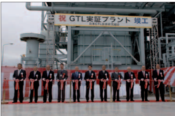
This plant in Niigata started up in April to test and verify the Japan GTL process.
