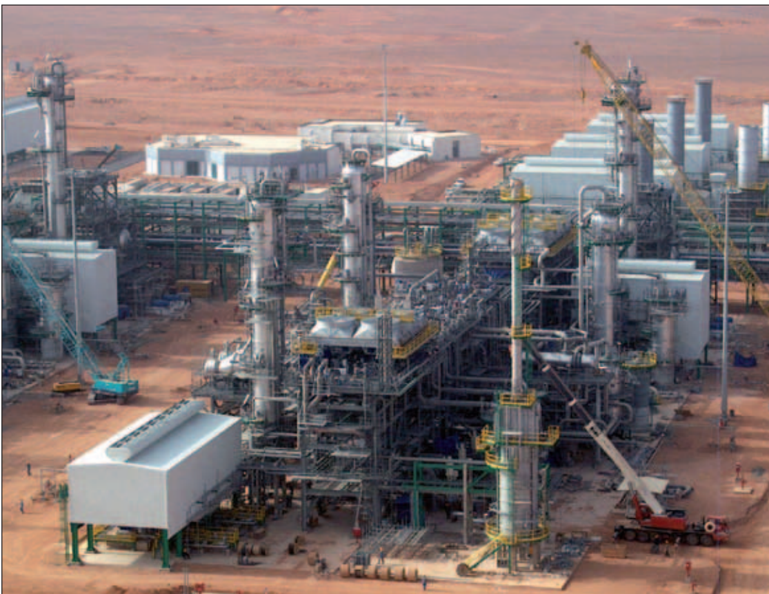
The Wafa gas treatment plant.
