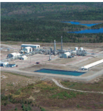
Sable Gas Plant, adjacent to LNG site, Goldboro, Nova Scotia.
