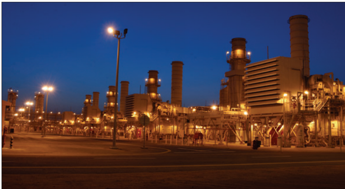
The Middle East will play an ever more important role as a supplier of natural gas. The picture shows the Haradh gas plant in Saudi Arabia.
