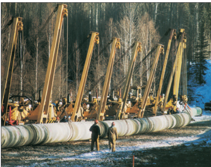
Pipeline integrity is a vital issue.
