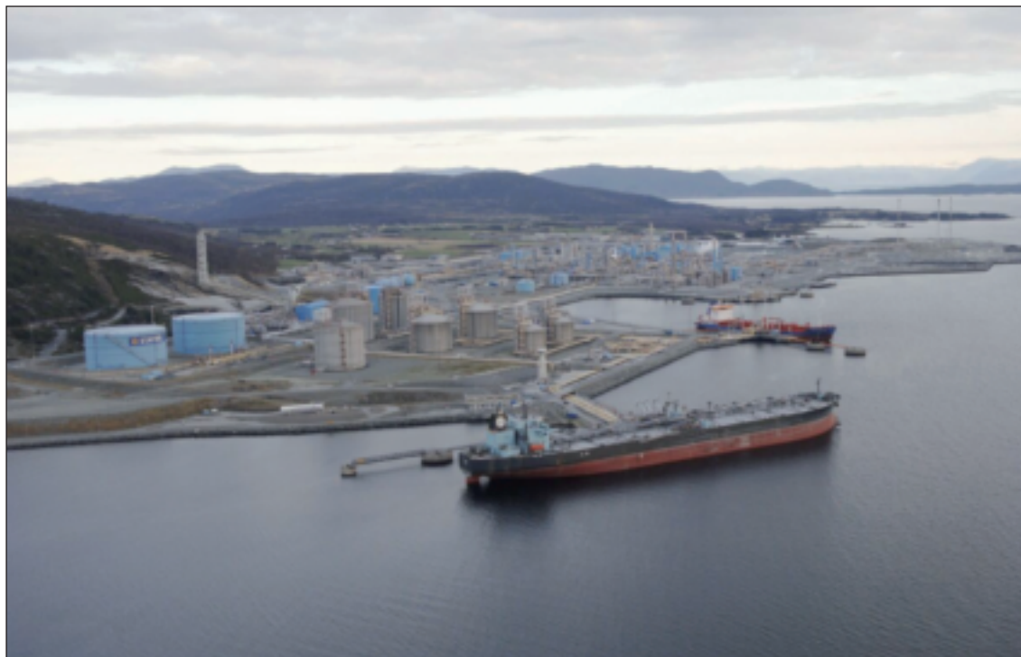
PGC A's second meeting included a technical visit to the gas processing plant at Kårstø.
