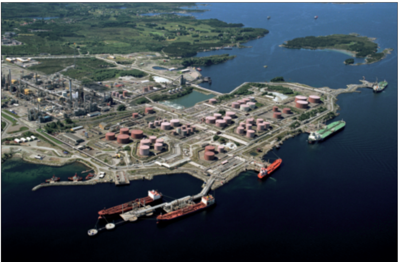
The modernisation of the Mongstad refinery is one of Norway's biggest energy efficiency projects.
