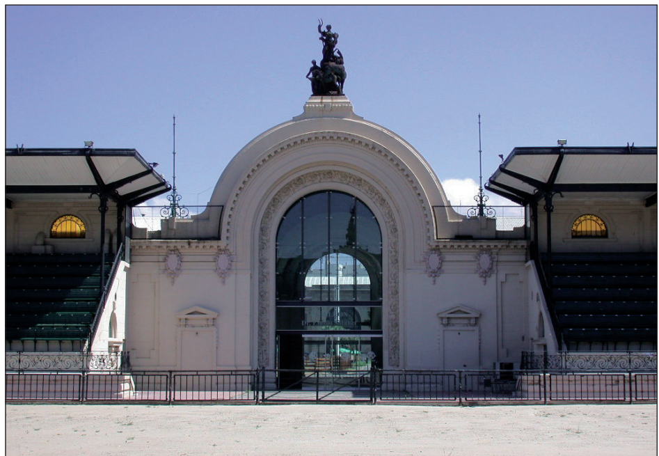
La Rural Congress & Exhibition Centre (ABOVE) will be the venue for WGC 2009. The floor plan is shown on page 56.
